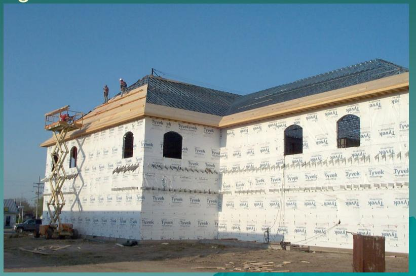
VT unfading green slate was installed on the yellow pine decking with stainless steel nails. This roof could last 200 years.
