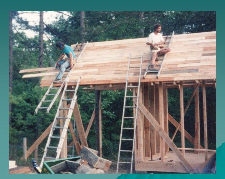
Planed, kiln-dried lumber is also commonly used. Yellow pine boards are shown here being installed on a bank.
