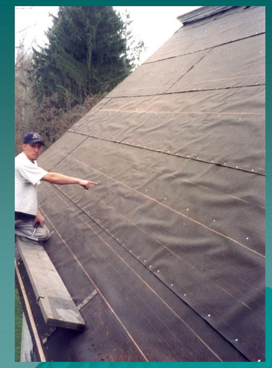
Smooth-shank copper nails are commonly used. Stainless nails may be needed on harder decking material
